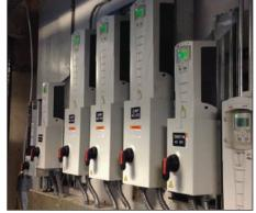
Installing VFDs (above) and some new compressors (below) helped increase system performance.
